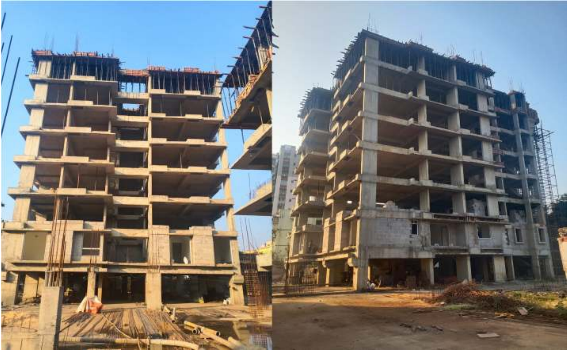
BLOCK 2- 8 th floor slab casting 2/3 flat completed rest work in progress.
